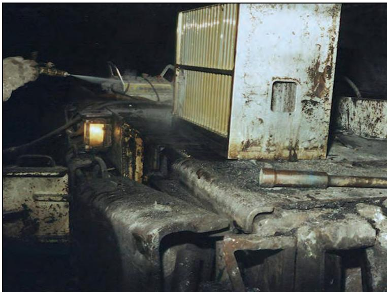
Figure 4-8.—Cleaning the demister with a water nozzle.
