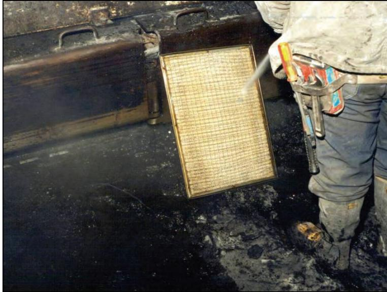
Figure 4-7.—Cleaning scrubber filter panel with water spray.
