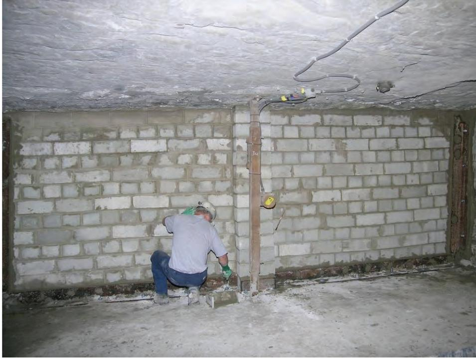
**Figure B-31.—Mortar filling the gaps between the steel angle hitching and the blocks along the floor and ribs.**
