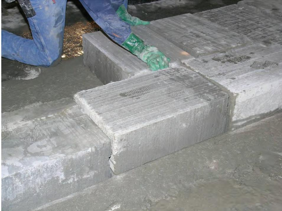
**Figure B-24.—Positioning the Omega blocks in a staggered pattern for the first course.**
