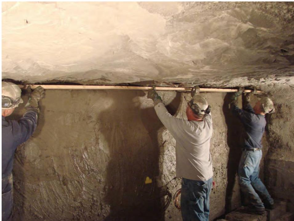
**Figure B-27.—Installing the crossboard on the outby side of C-drift seal.**
