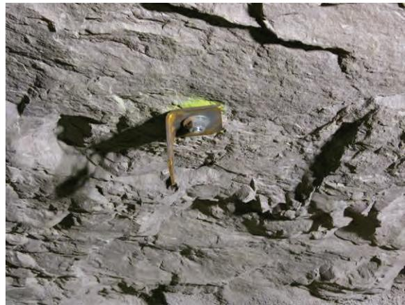
Figure 6.—Roof plates and belt hanger at 234 ft from the face.
