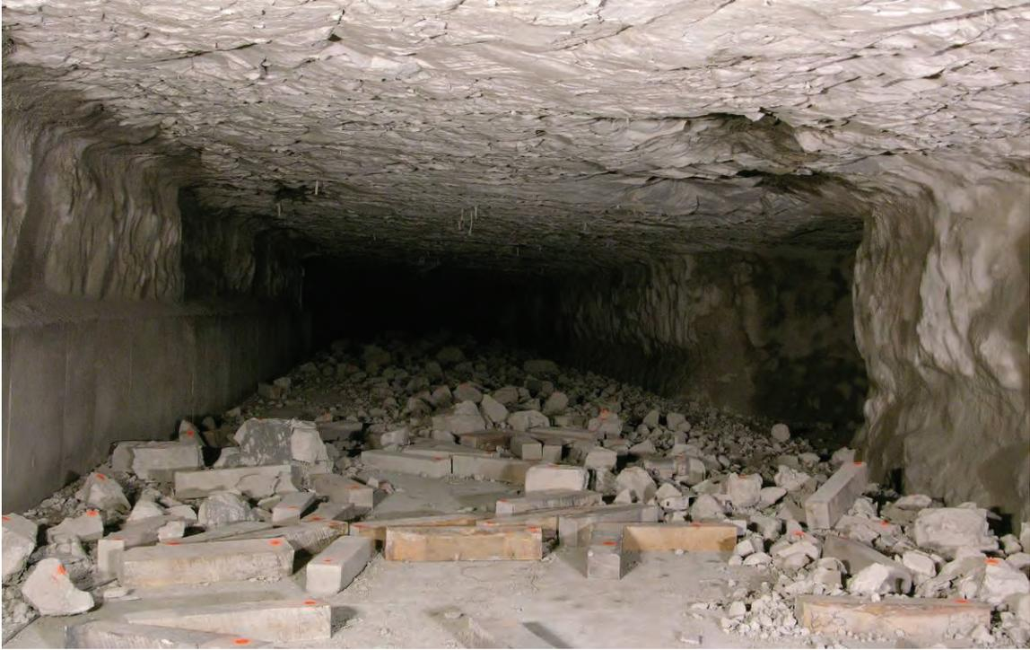
**Figure 47.—Debris from C-drift seal, stopping, and wood cribs looking outby from 403 ft.**
