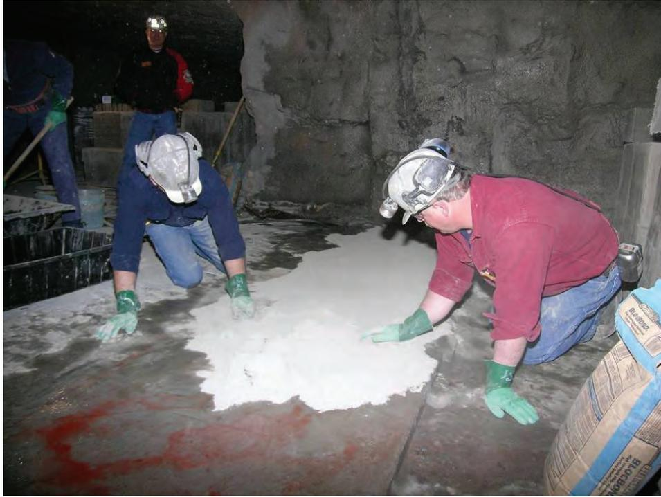
Figure B-10.—Dry BlocBond being spread to a 0.5-in-thick layer on the dampened concrete floor in X-3.
