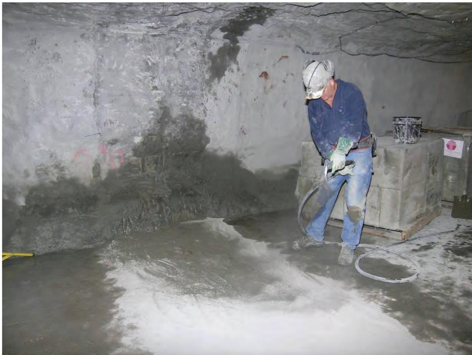
**Figure B-23.—Wetting the dry layer of BlocBond with a fine spray of water.**
