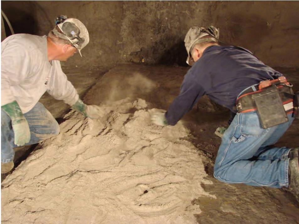
**Figure B-18.—Applying the 1.5-in-thick layer of dry BlocBond to the dampened concrete floor in X-3.**
