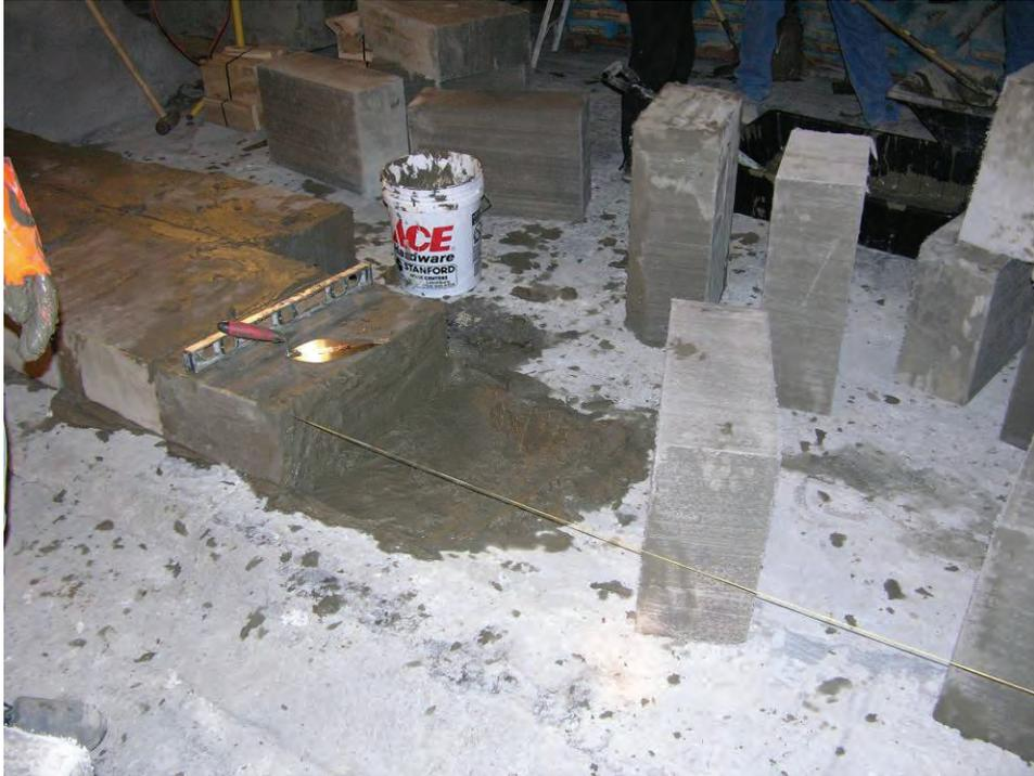
**Figure B-1.—BlocBond applied to concrete mine floor.**
