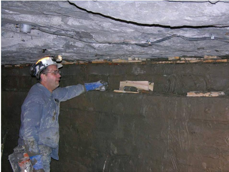
**Figure B-8.—View from the C-drift side showing the rough-cut lumber wedged between the mine roof and blocks across the center of the seal.**
