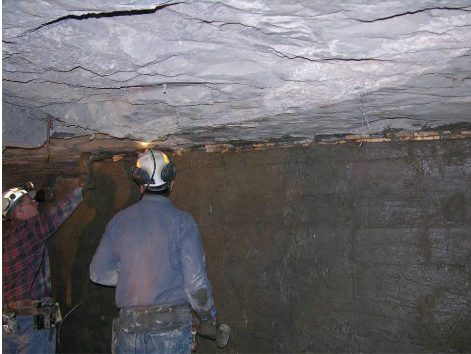
**Figure B-7.—One row of wood placed flush with the edge of the blocks on the B-drift side.**
