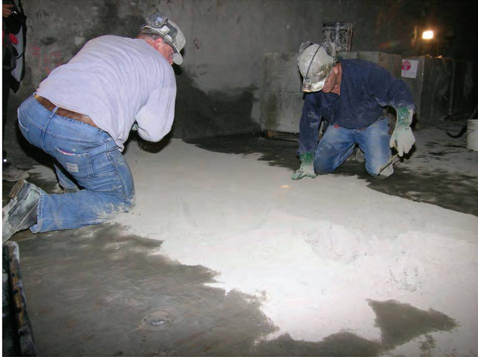
**Figure B-22.—Applying a 1.5-in-thick layer of dry BlocBond on the dampened concrete floor across C-drift.**
