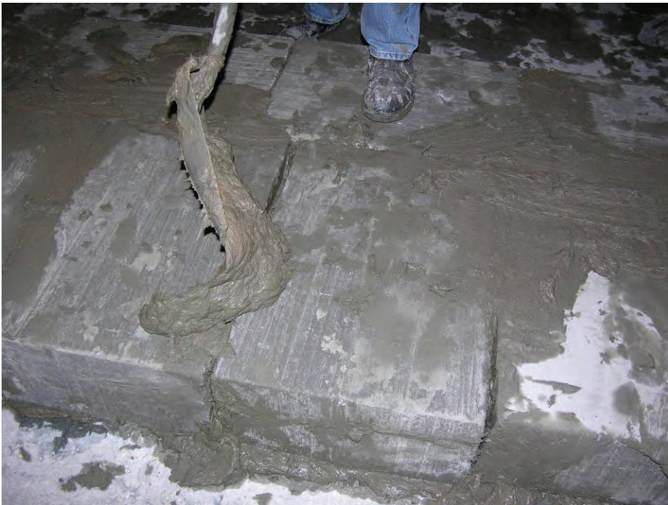
**Figure B-2.—BlocBond being applied to gaps between the Omega blocks.**
