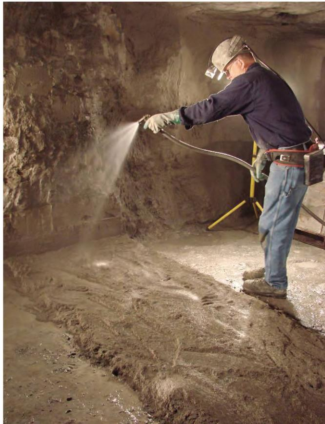
**Figure B-19.—Applying a fine water spray to the dry BlocBond layer.**
