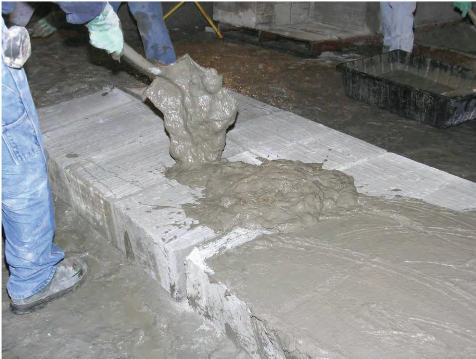
**Figure B-20.—Applying the properly mixed BlocBond to the first course of Omega blocks.**
