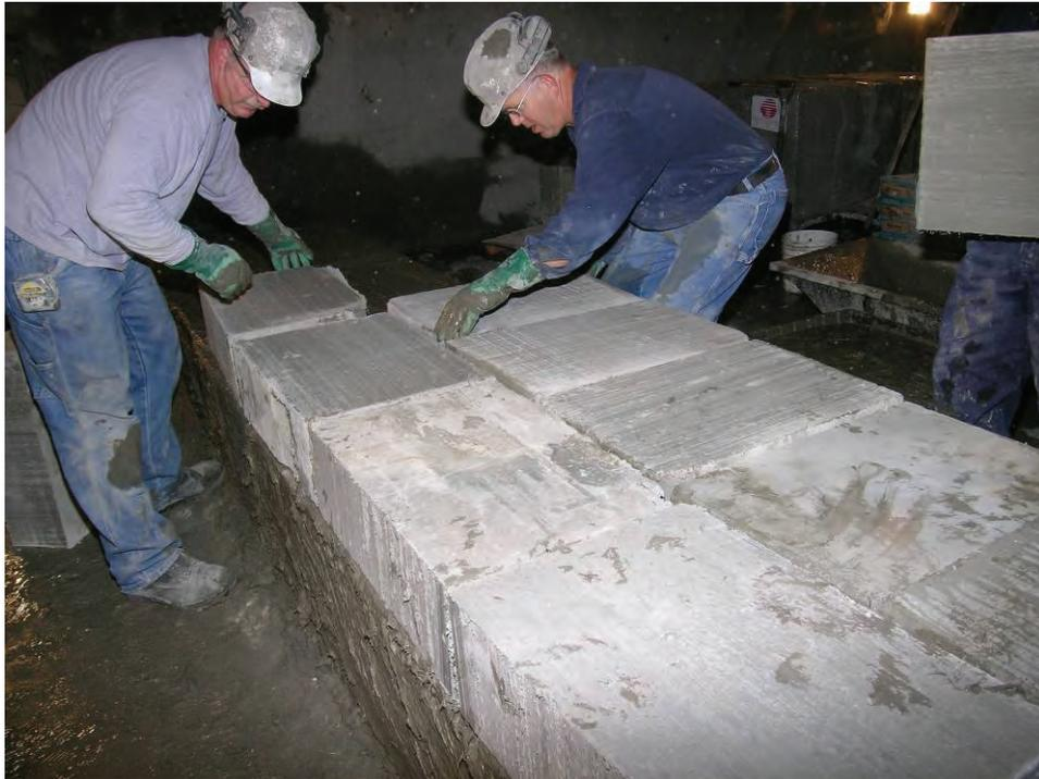
**Figure B-26.—Positioning the second course of Omega blocks in a transverse pattern.**
