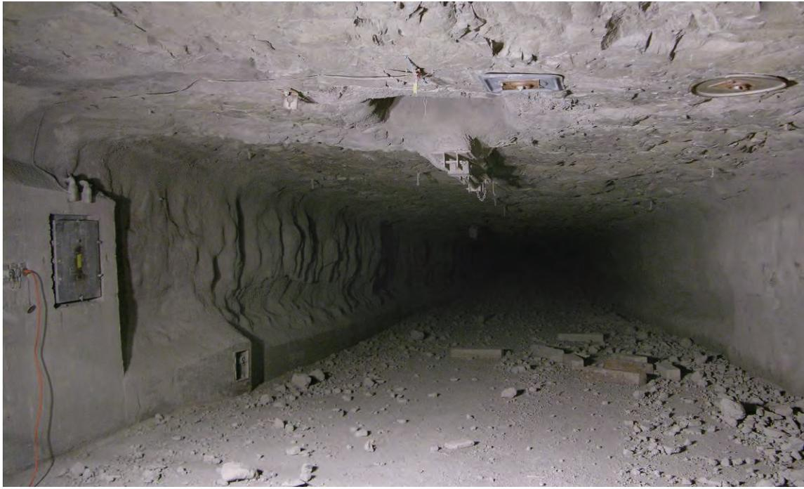
**Figure 70.—Debris in C-drift after Test 6 (LLEM #506) looking outby from 757 ft.**
