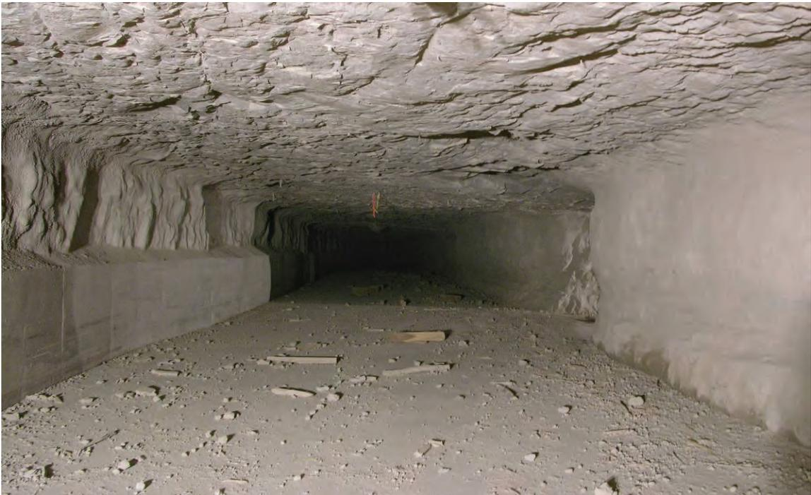
**Figure 67.—Debris in C-drift after Test 6 (LLEM #506) looking outby from 403 ft.**
