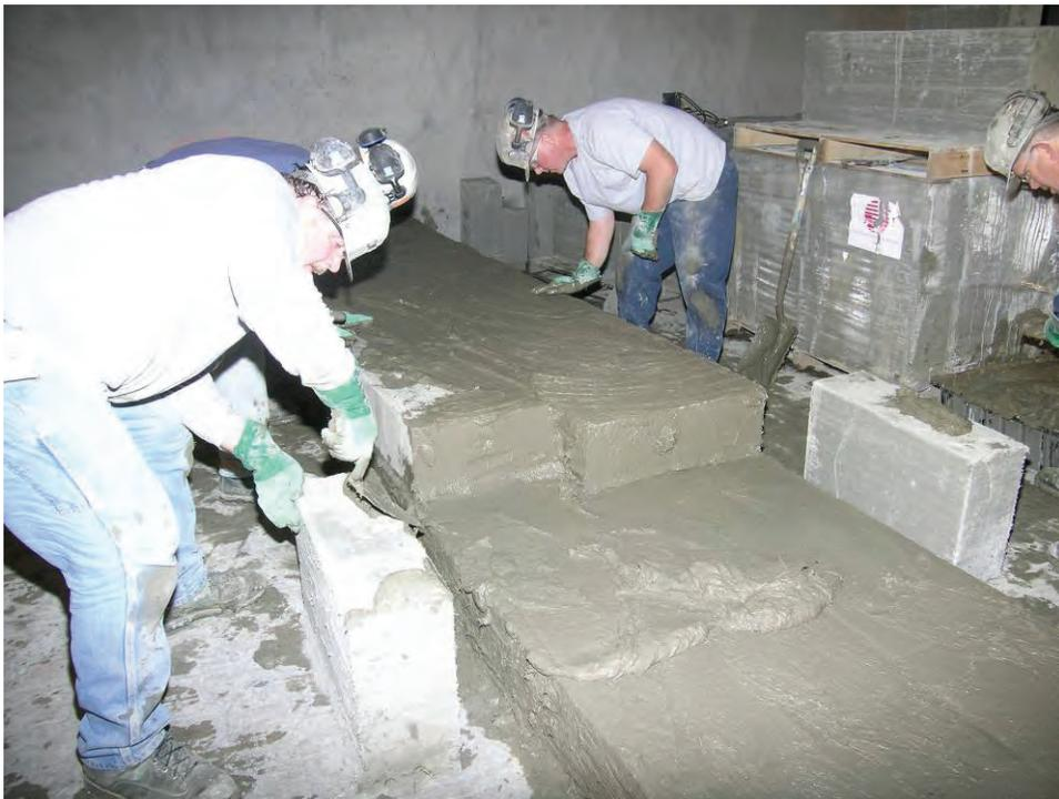
**Figure B-15.—Omega blocks laid wet with fully mortared (BlocBond) horizontal and vertical joints.**
