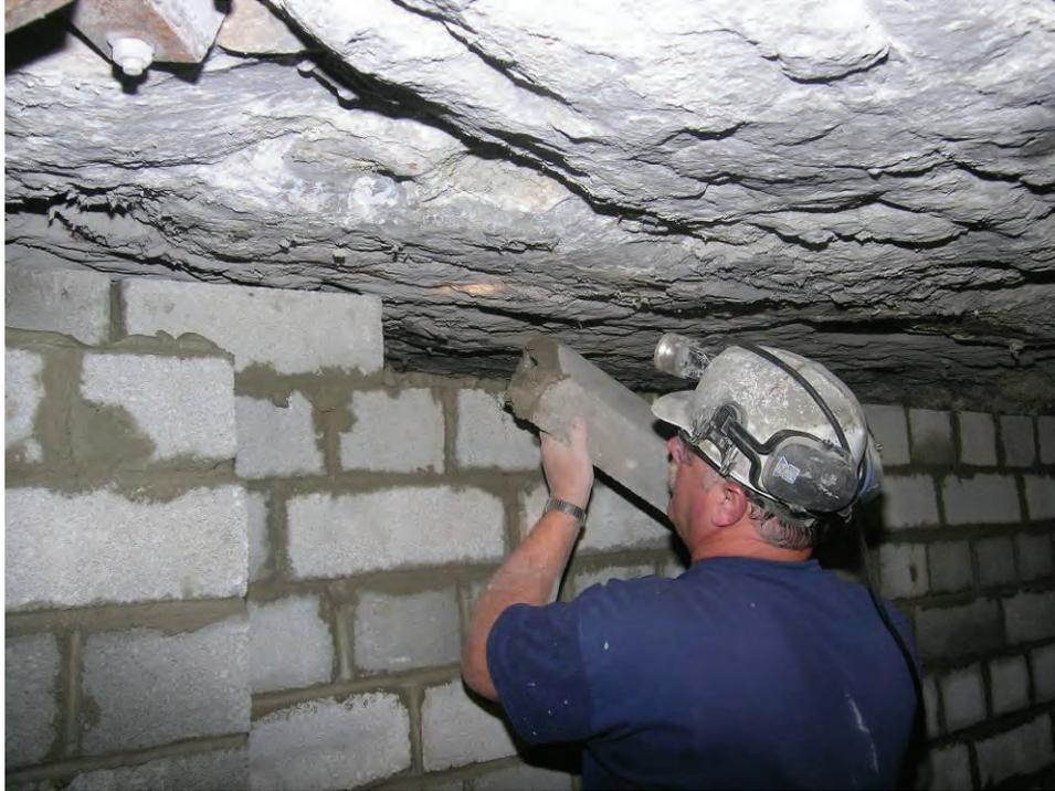
**Figure B-29.—Installing cut blocks on top course.**
