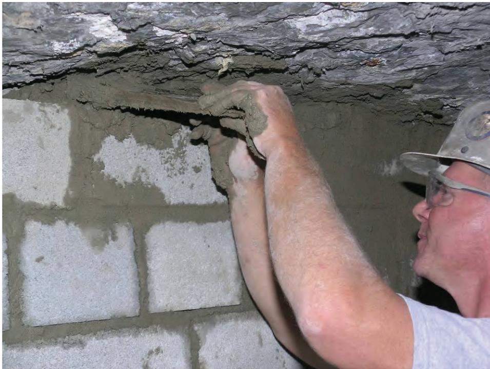
**Figure B-30.—Completely filling the gap between the top course of blocks and the mine roof with mortar. The blocks were not wedged.**
