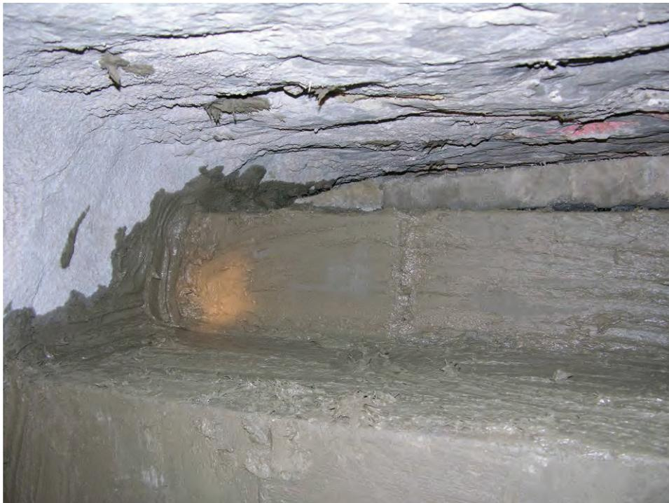
**Figure B-6.—View of top portion of seal from C-drift side after B-drift side was completed. The last two block courses and middle and inby crossboards were installed from the C-drift side to complete the seal.**
