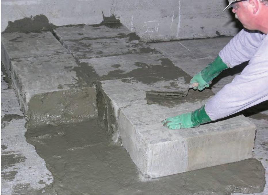
**Figure B-14.—A 0.25- to 0.5-in-thick layer of properly mixed BlocBond on the floor.**
