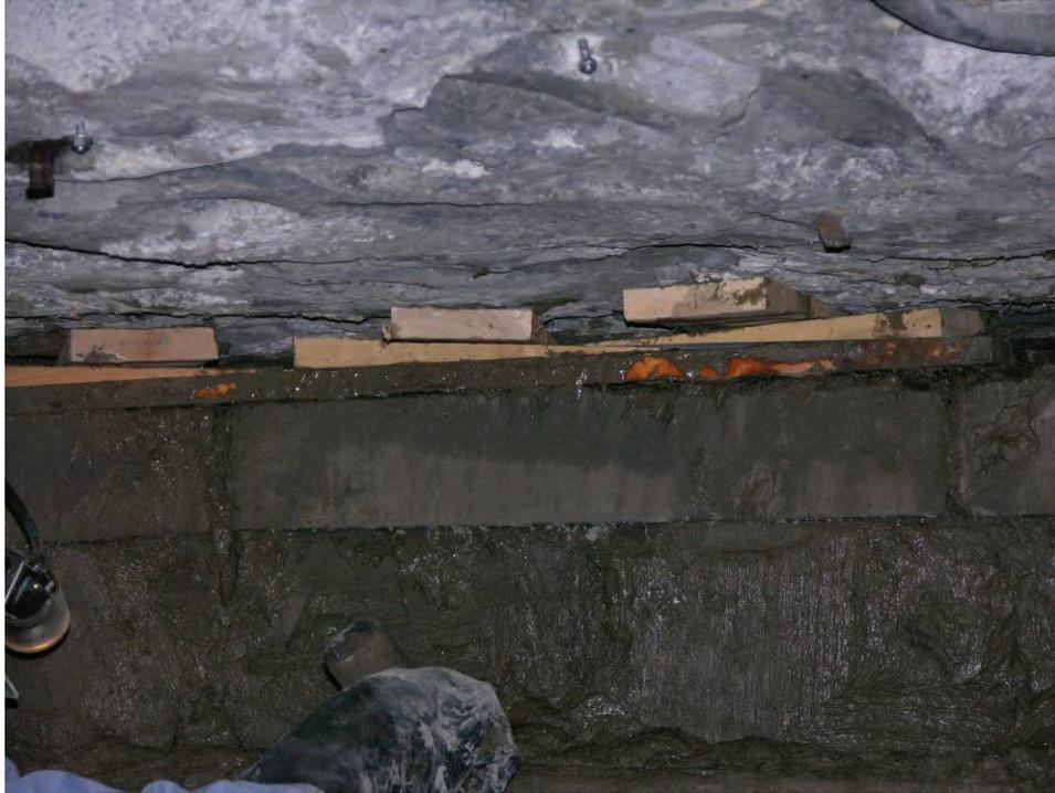
**Figure B-9.—Closeup of the wood wedges, installed between the mine roof and the rough-cut board, used to tighten the Omega block seal.**
