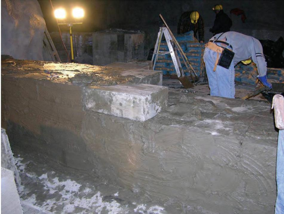
**Figure B-3.—As each Omega block course was completed, BlocBond was also coated on the exposed B- and C-drift sides of the blocks.**
