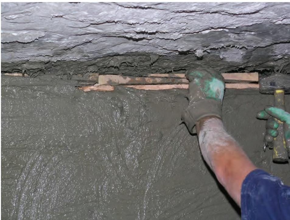
**Figure B-21.—Driving the wedges (skin to skin) between the crossboard and mine roof.**
