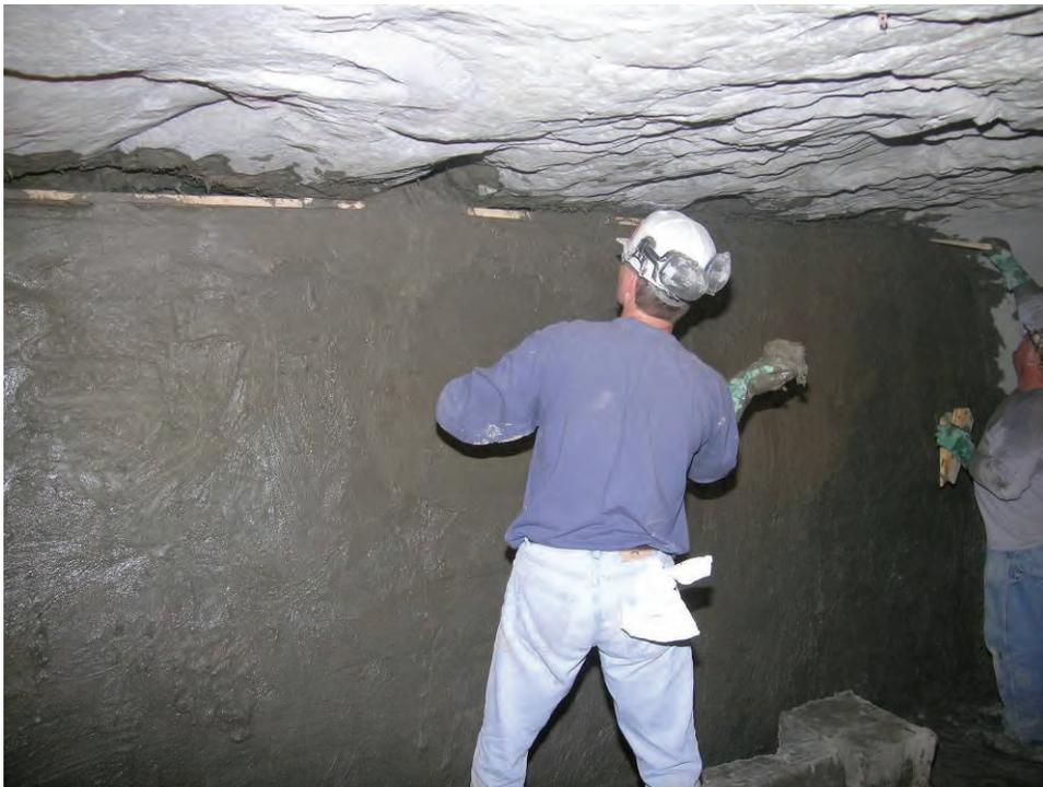
**Figure B-17.—Hand slinging the BlocBond to fill the gaps between the previously installed center board and the outby board.**
