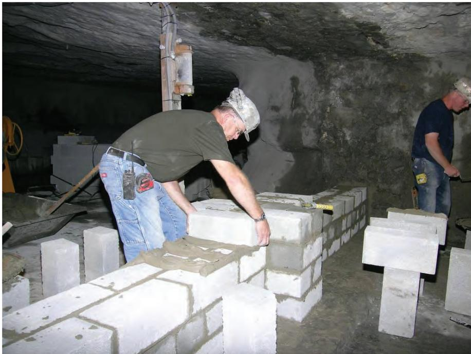
**Figure B-28.—Full wet-bed construction on all horizontal and vertical block joints.**
