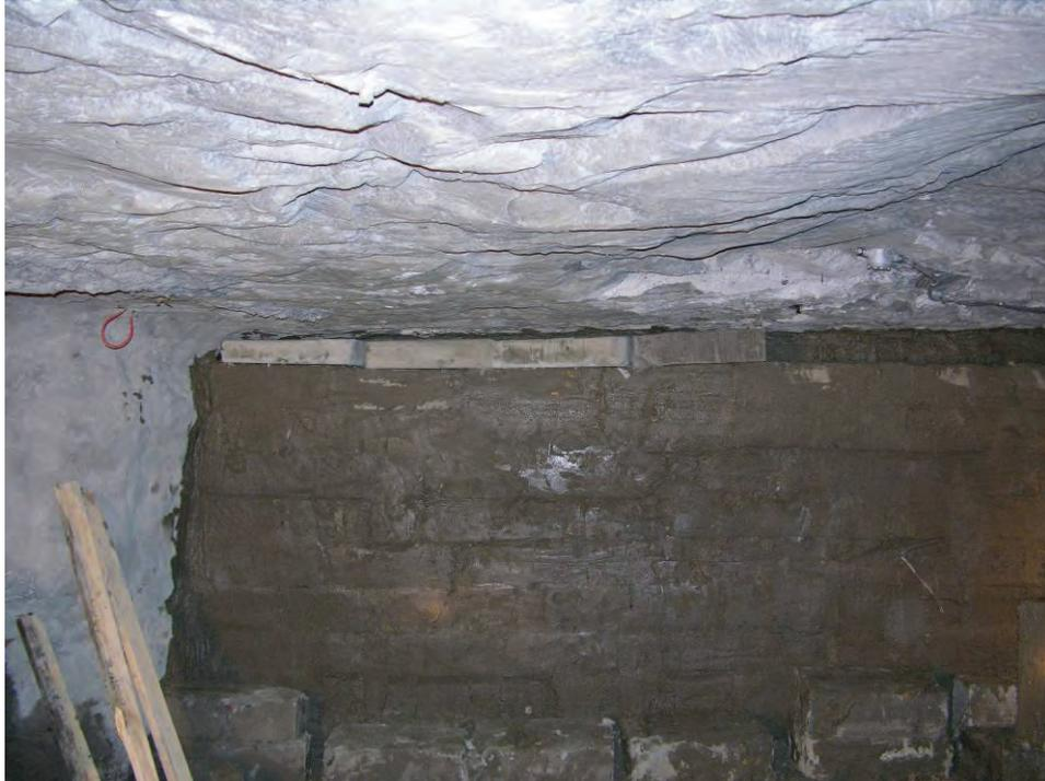
**Figure B-5.—Cut blocks on top course to provide 2-in gap to roof.**
