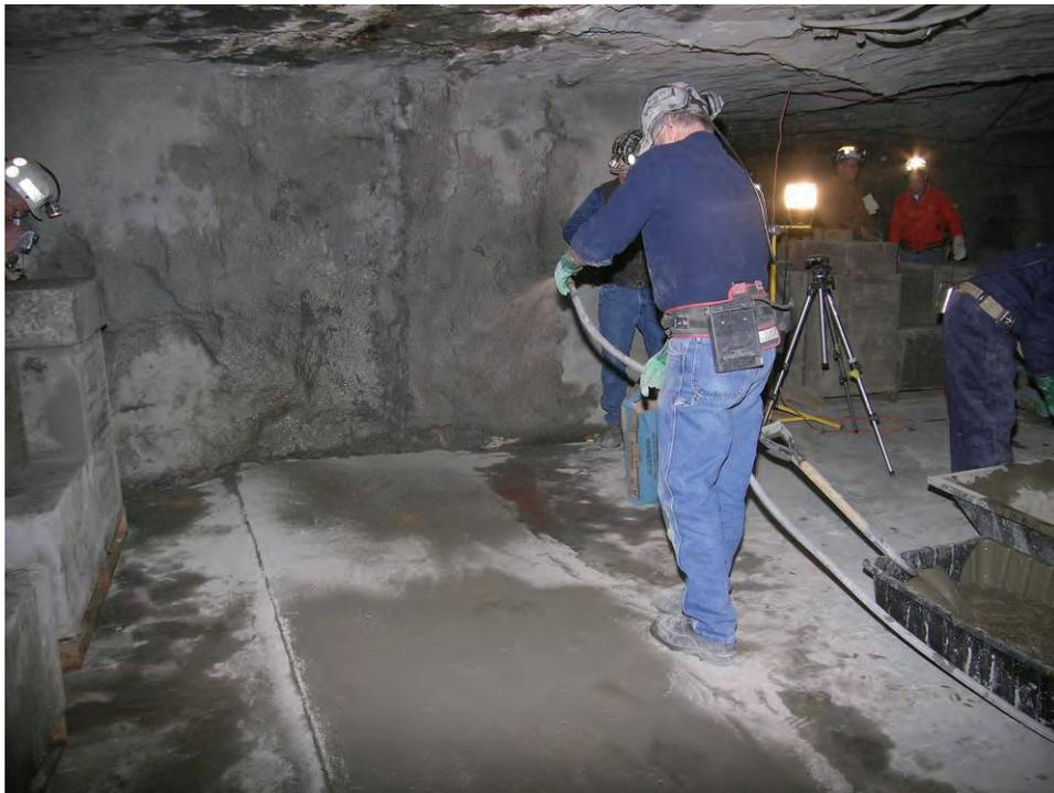
Figure B-11.—Wetting the dry layer of BlocBond before positioning the Omega blocks.
