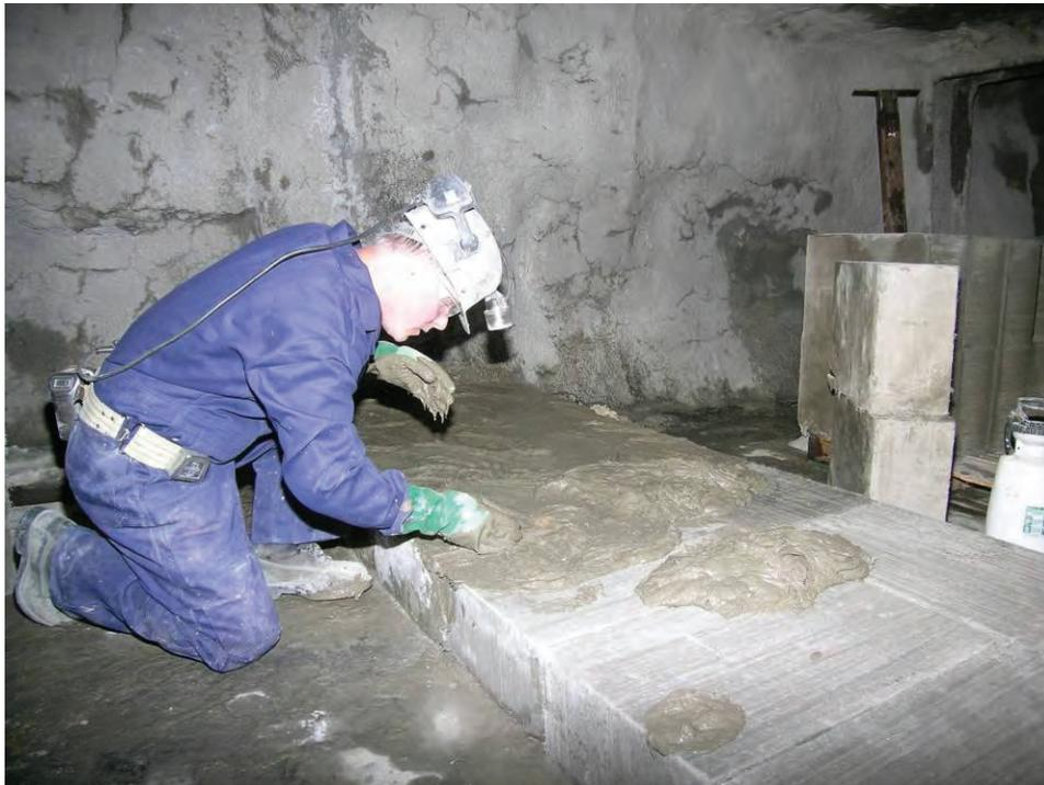
**Figure B-13.—Applying BlocBond to the top of the first course. The BlocBond is forced into the vertical joints using only gloved hands.**
