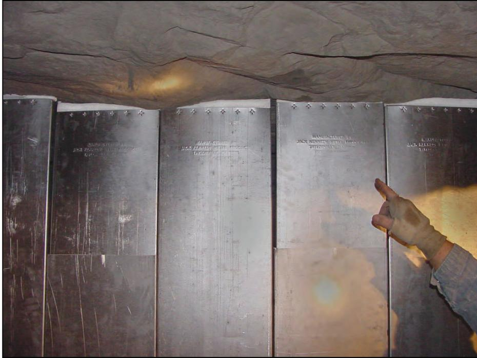
Figure 17.—Polystyrene foam head seal used to provide enhanced closure between metal panel and roof, as viewed from the C-drift side.
