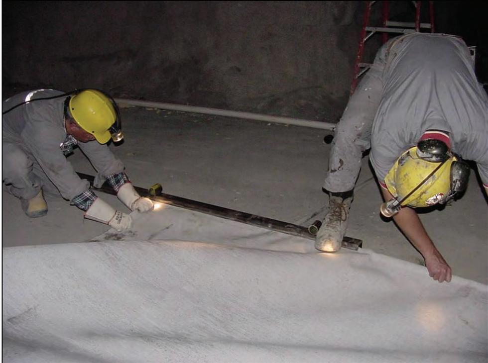
**Figure 26.—Inserting pipe/sleeve into top box section.**
