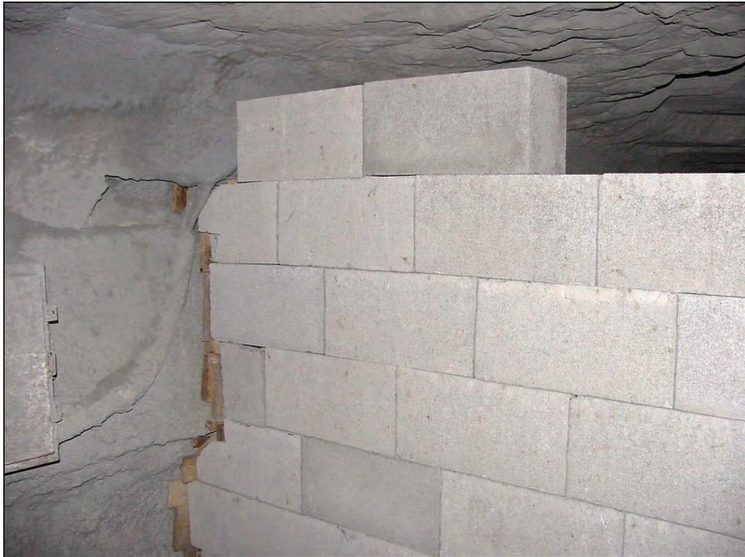
**Figure 3.—Dry-stacked hollow-core concrete block stopping construction, with staggered joints.**
