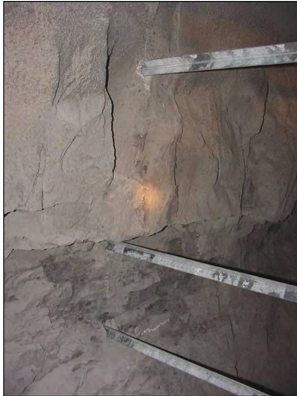
**Figure 15.—Three horizontal steel angles inset into rib.**
