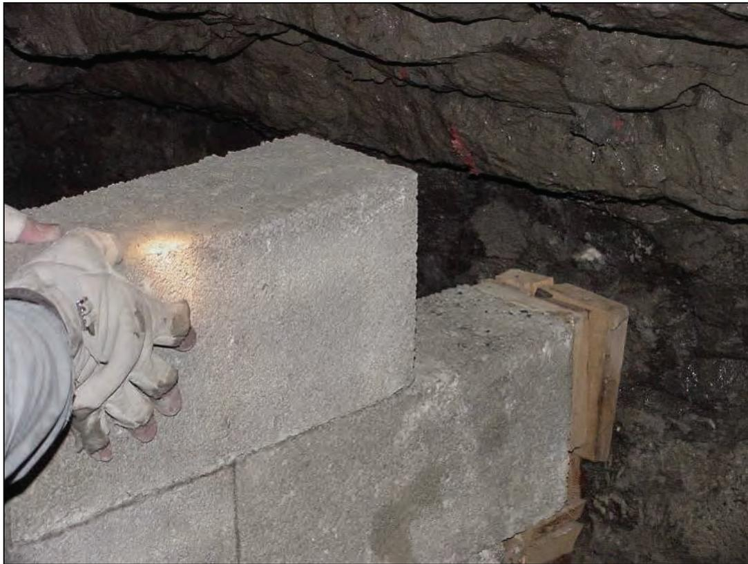
**Figure 8.—Dry-stacked solid-concrete-block stopping construction with staggered joints.**
