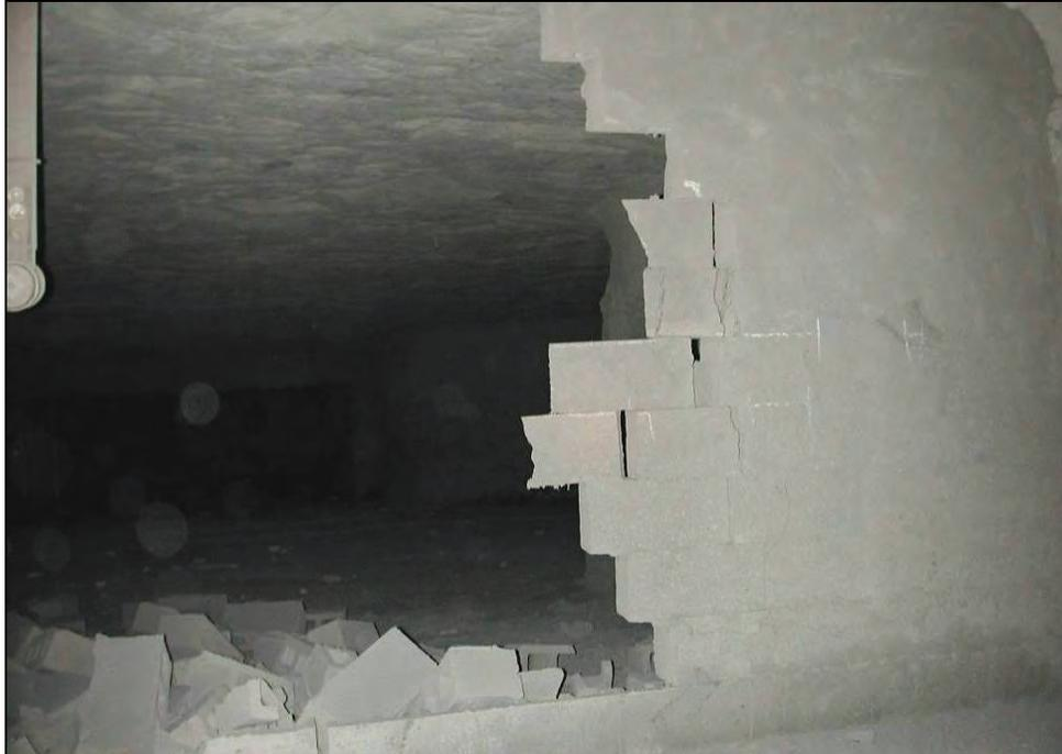
**Figure 58.—Additional blocks partially dislodged from the right side of X-6 dry-stacked hollow-core concrete block stopping after test #434, viewed from C-drift.**
