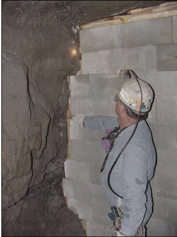
**Figure 9.—Wood wedges between the stopping and rib for dry-stacked solid-concrete-block stopping.**
