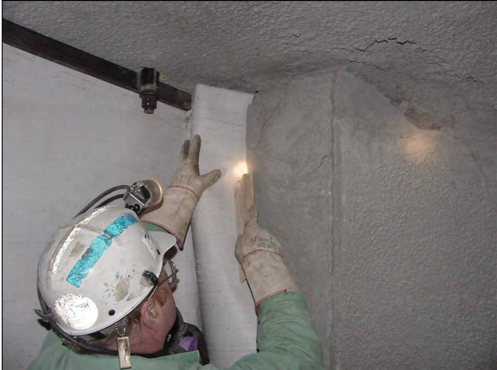
**Figure 28.—Wedging woven cloth into mine rib.**
