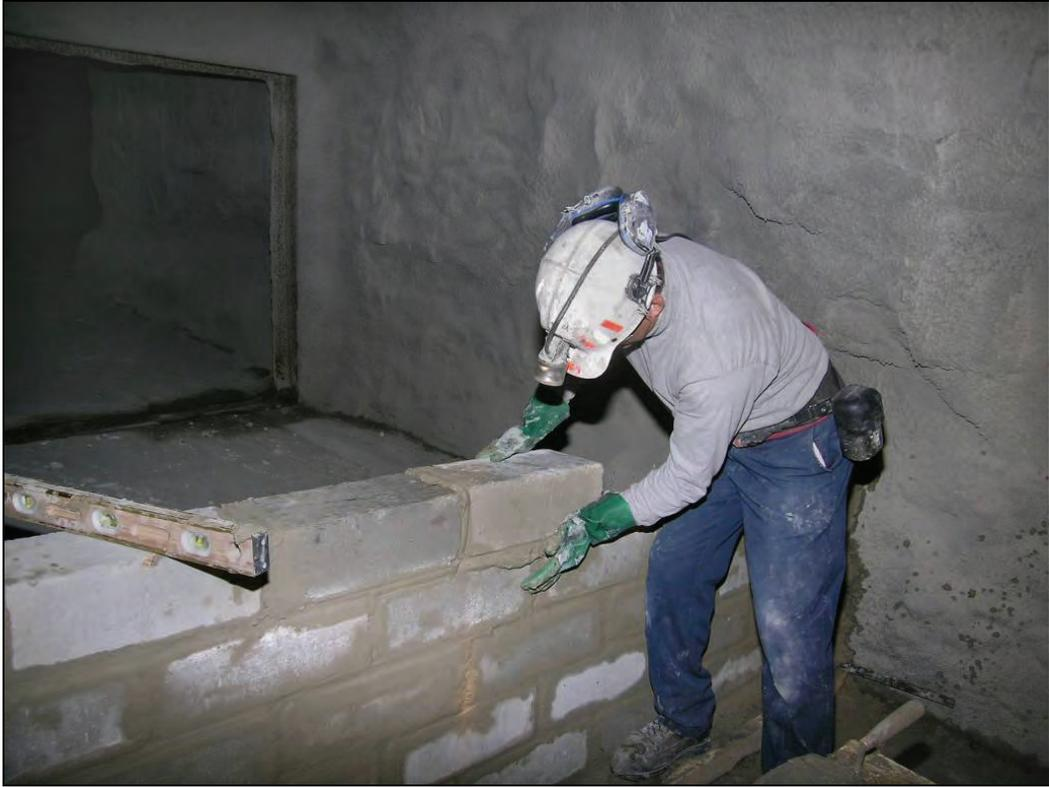
Figure 12.—Wet-laid solid-concrete-block stopping construction with staggered joints.
