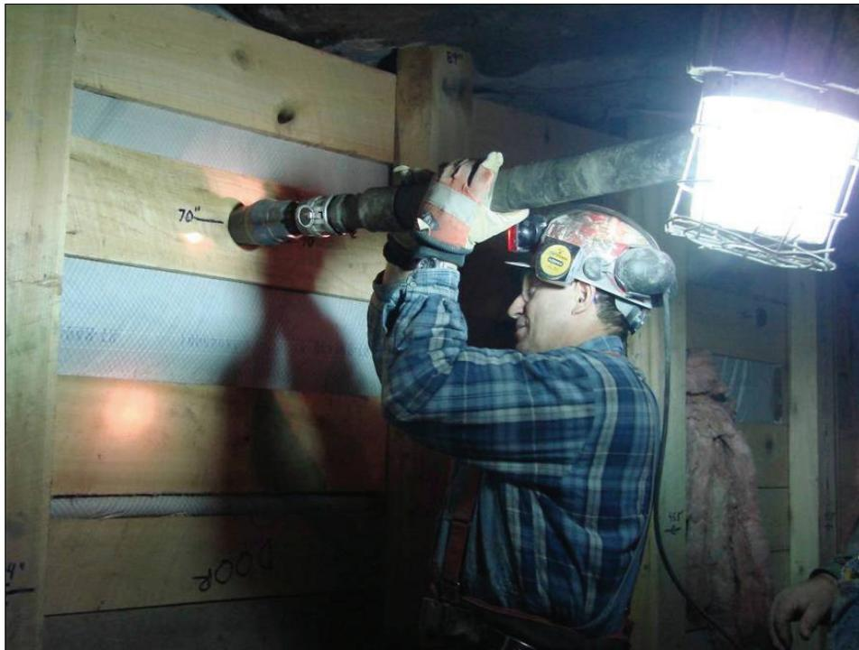
**Figure 11.—Connection of the slurry injection hose for filling the top third of the seal.**
