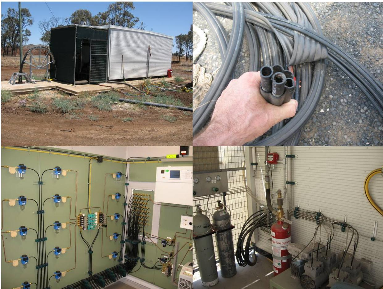
**Figure 8.—Continuous atmospheric gas monitoring system in Australia. Top left: Monitoring shed over mine showing borehole and sample tubes. Top right: Close-up of sample tube bundle. Bottom right: Sample tube pumps. Bottom left: Inside monitoring shed showing manifold and gas analyzer.**
