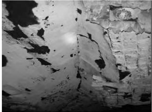
**Figure 1.—Roof fall initiated by unfavorably oriented slip planes.**
