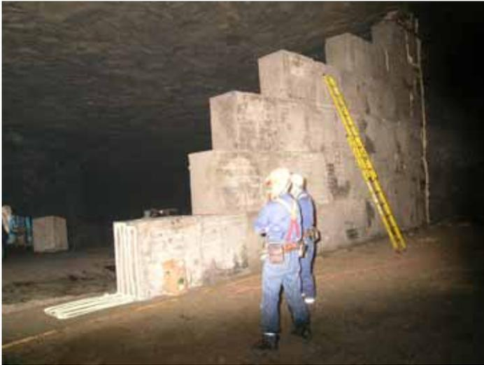
Figure 2.—Partially constructed Super Stopping.
