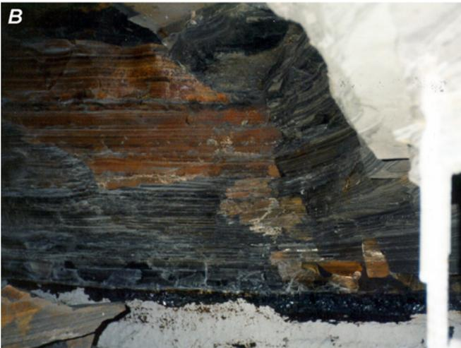
Figure 36.—Roof fall terminating against a large joint face. A, Diagram; B, photograph.
