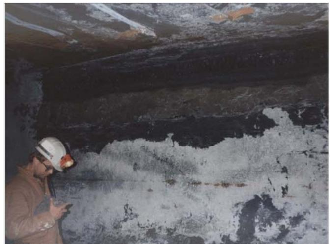
Figure 10.—As a weak seat earth thickens in a southern West Virginia mine roof, it causes roof bolts to miss anchorage in a strong sandstone.
