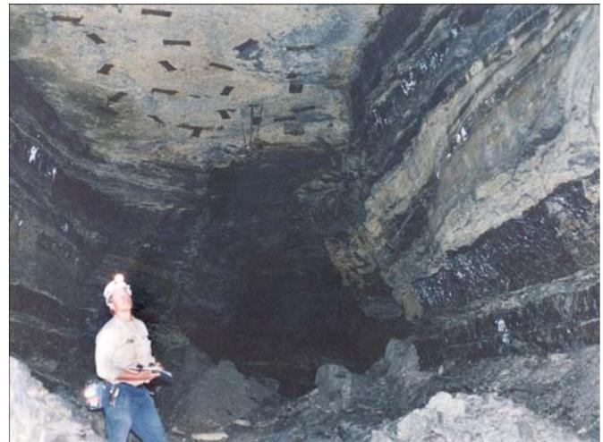
Figure 14.—Rider coalbeds above the main bench of the Pittsburgh Seam.
