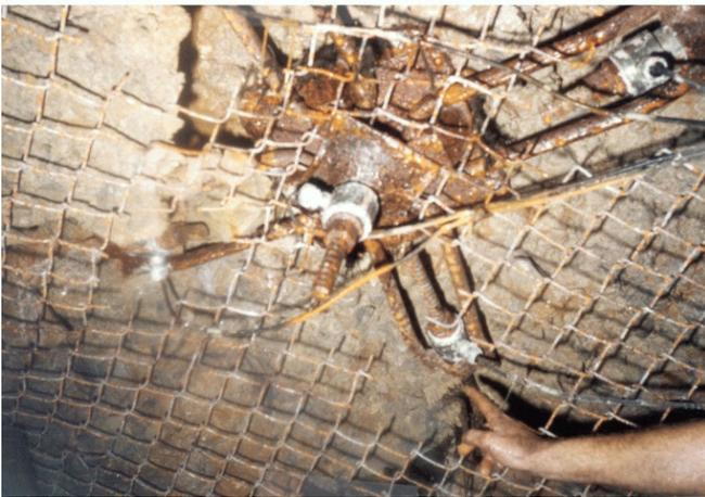
Figure 17.—Load cells at truss four-way bracket.
