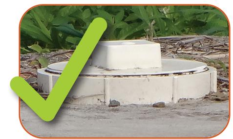
Septic tank sealed with PVC cap
