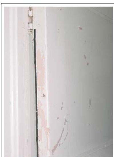
FIGURE 5.7 Impact surface on door and frame.
